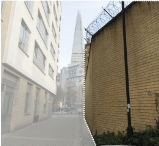
1 Southall Place - site bounded by blank barbed wall
