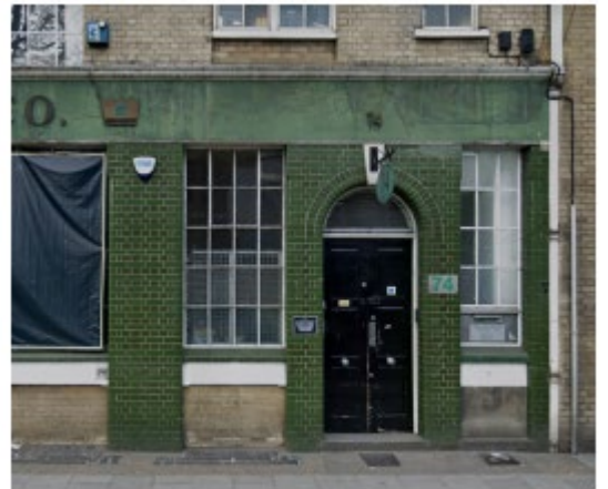
6 Elevation of the warehouse building showing the distinctive green glazed brick facade
